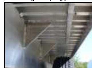
Cargo Wench tie bar under deck
