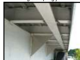
Under deck tie bar
